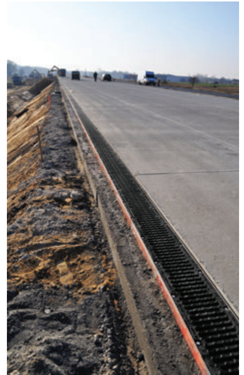
Expressway S8 Zawada AS-200 - 900 LM
