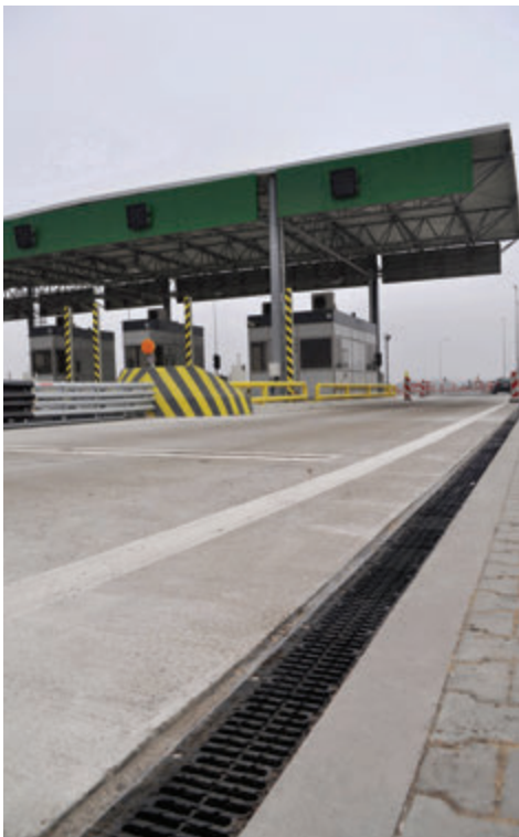
Motorway A2 Buk AS-150
