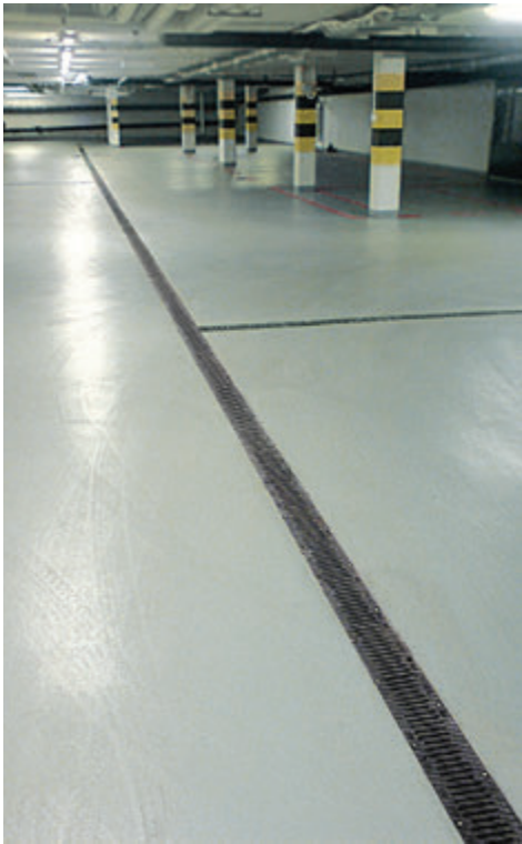
Underground garages AS-A100
