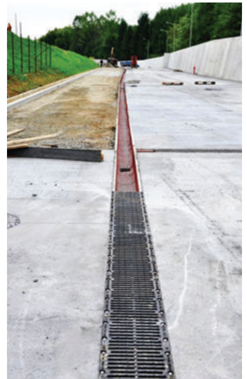
Municipal Landfill Site Barycz AS-300 - over 700lm
